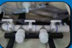
Solar/Gas/Heat Pump Connections in Place
